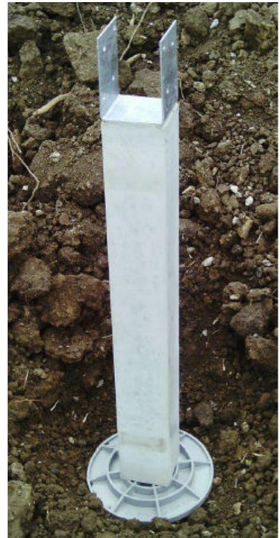
Figure 9.1: Deck Post on AG-CO Molded Plastic FootingPad
